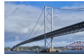
Forth Road Bridge
